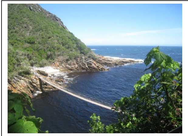
Storm Mouth Suspension Bridge, South Africa, sent by Ida Eisses, TC 31 Walsrode, Germany
